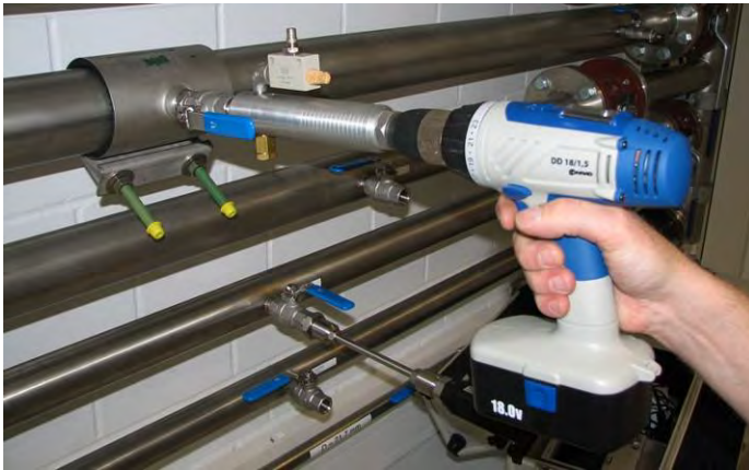
Drilling with CS drilling jig Order no. 0530 1108
