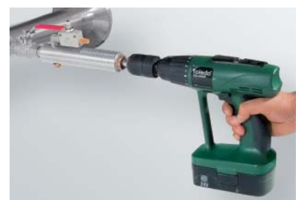
• Drilling under pressure
