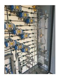
IPP built and installed a Hydrogen distribution system, tested at 650 bar. Most of the components came from the IPP portfolio:
